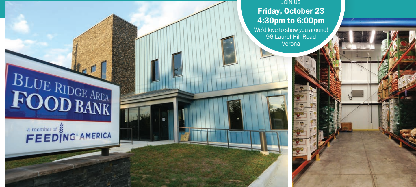
The Food Bank thanks our construction partners at Neilsen Builders
